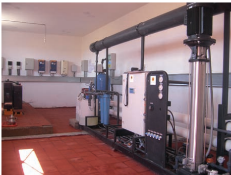
Figure 3. Photographs of the RO unit and the PV panels for the Benhassine site.
