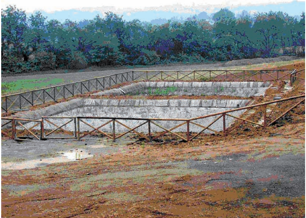
Figure 1. The constructed wetland realized near Sellustra stream.
