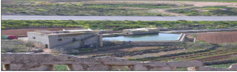
Fig. 5. Typical uncovered reservoir in the Maltese countryside
