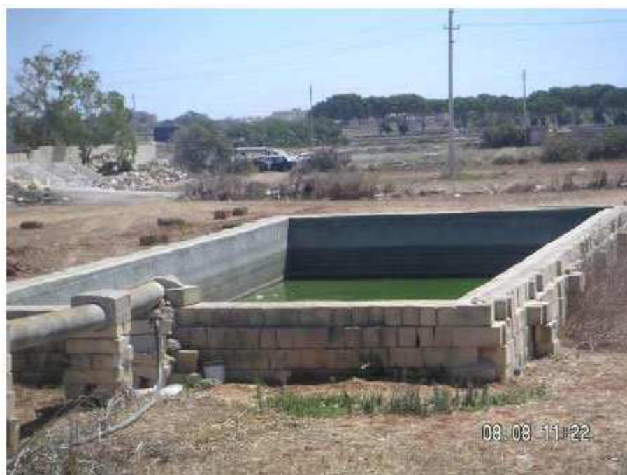
Fig. 1. Above ground water storage reservoir in Malta
