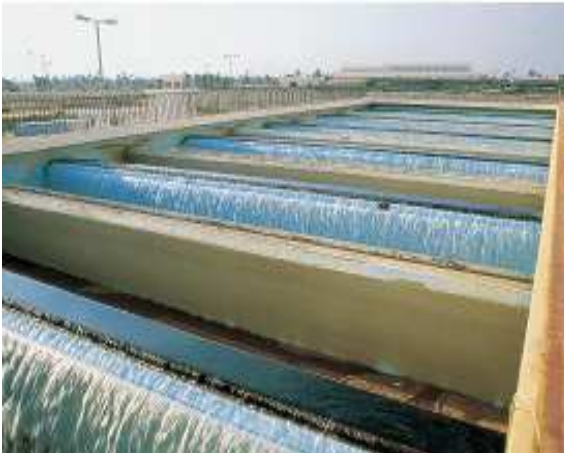
Figure 2: Water treatment plant.
