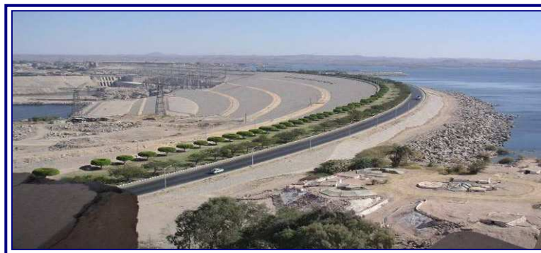
Figure 3: High Aswan Dam (MWRI, 2006).
