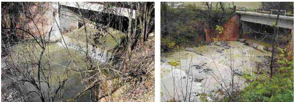
Figure 2. The slope built with stone blocks in order to smooth the drop under the bridge.
