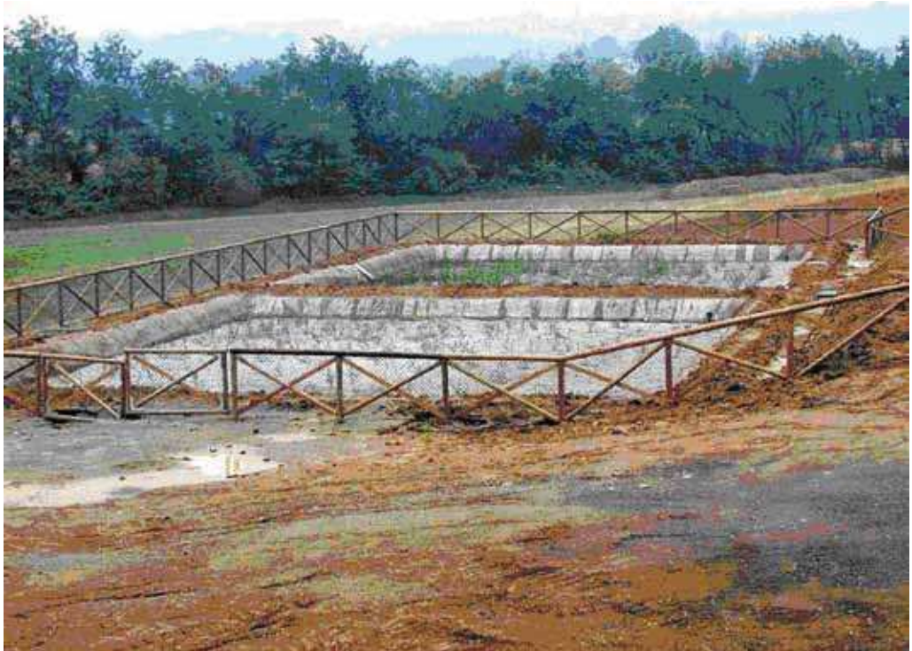
Figure 1. The constructed wetland realized near Sellustra stream.
