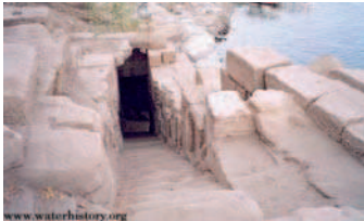
Figure 11. Staircases Nilometers descending into the Nile with marks indicating various levels.
