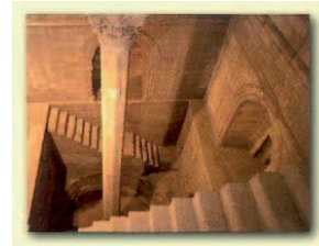
Figure 11. Staircases Nilometers descending into the Nile with marks indicating various levels.
